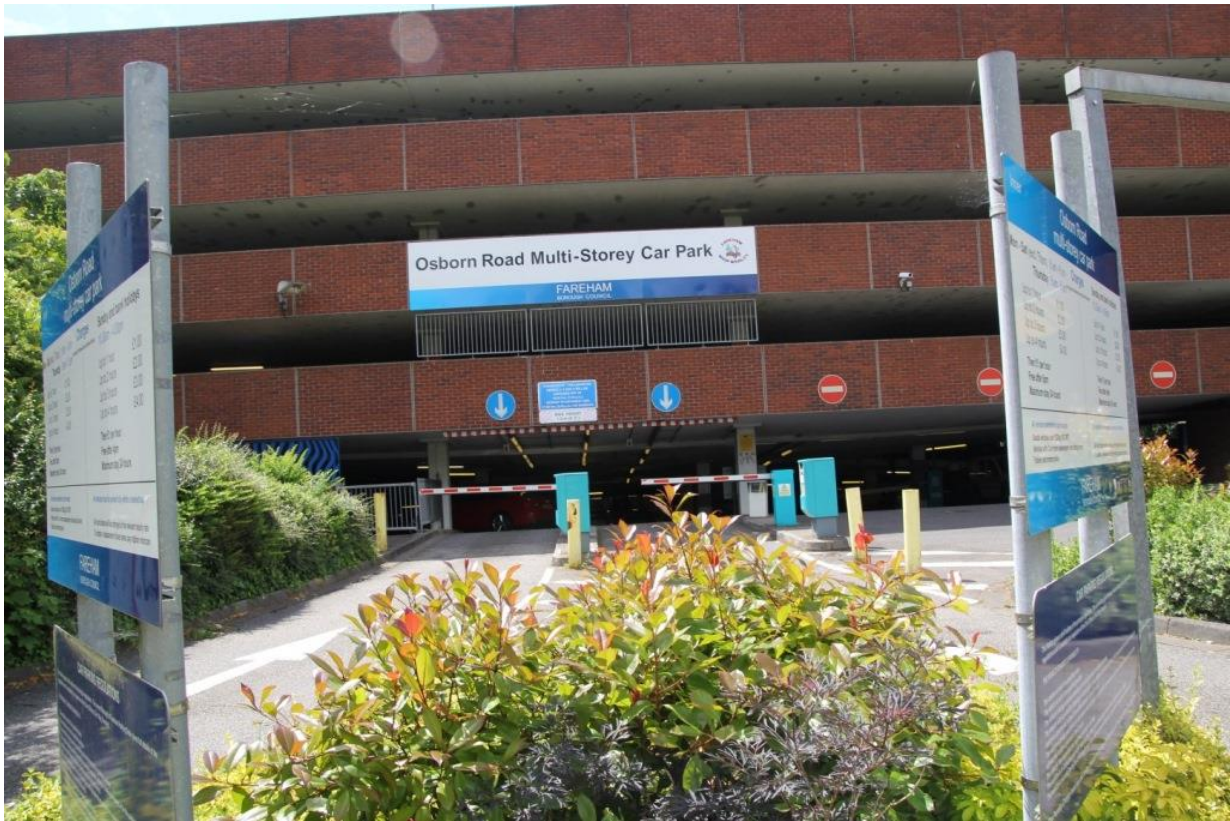
Osborn Road Multi-Story Car Park
